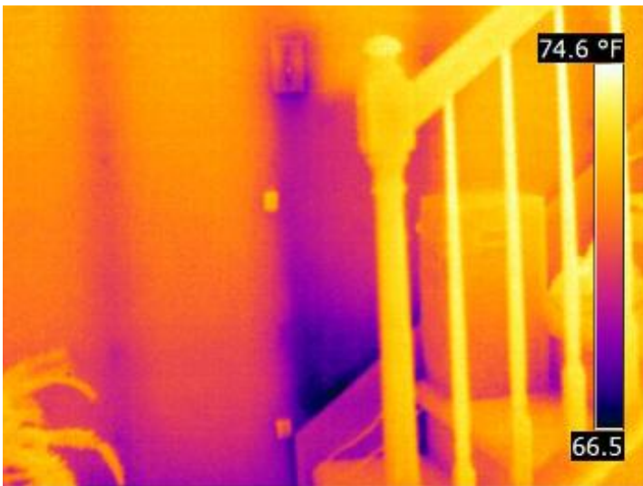
Air infiltration through the switch box from air infiltrating through the electrical service panel in the garage.
