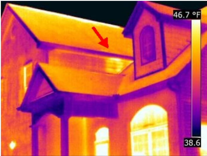
Inadequate insulation in the master bedroom is evident on the exterior wall of the house.
